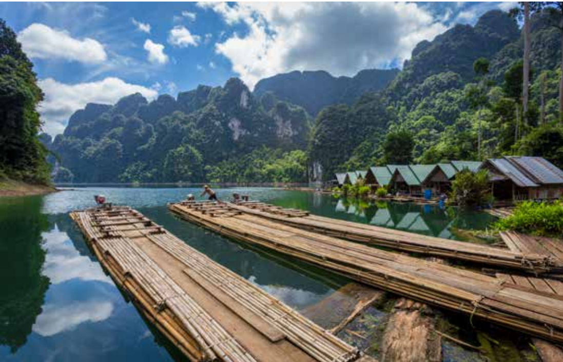
Rajjaprabha Dam or Chiao Lan Dam
