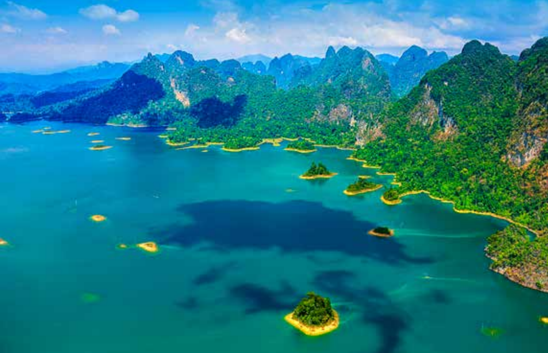
Rajjaprabha Dam or Chiao Lan Dam
