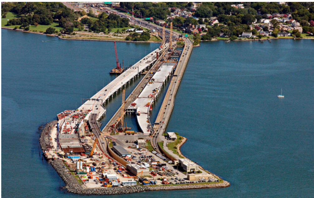
The Hampton Roads Bridge-Tunnel project (ที่มา: https://virginiabusiness.com/hampton-roads-bridge-tunnel-expansion-2027/ )
