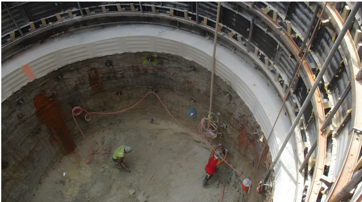
Big Creek Storage Tunnel
