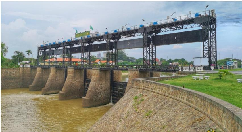
*Rama VI Barrage/Dam, which began construction in late 1915 and was completed in December 1924. Its function is to supply water to 680,000 Rai of agricultural land in every part of the Rangsit canal area.*
