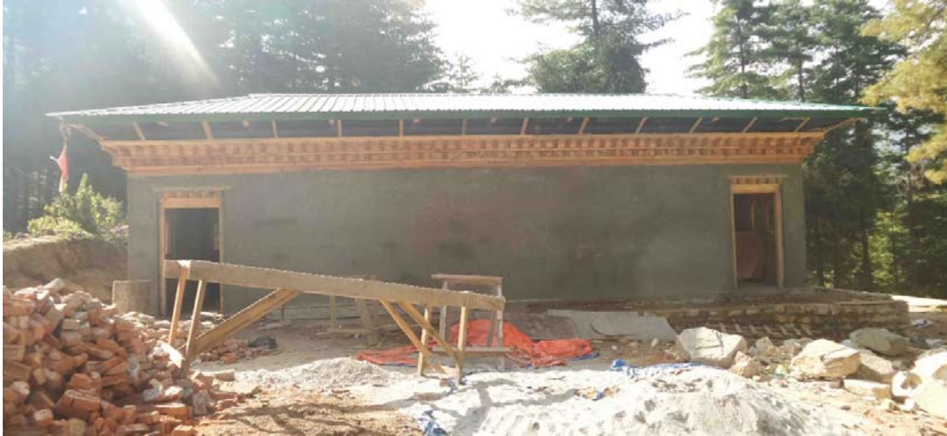
Figure Q1-12. Existing façade of Ramthangkha (Taksang base) restrooms construction
