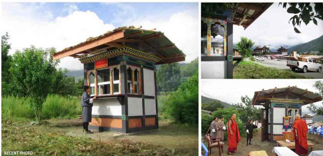
Figure Q4-24-26. Construction monitoring of Tashichho Dzong ticket booth.
