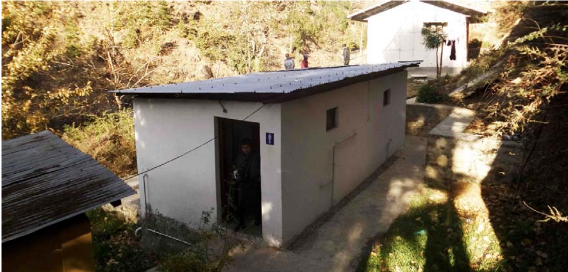
Figure Q1-46. Existing Chuzom restrooms ( Thimphu-Paro highway )
