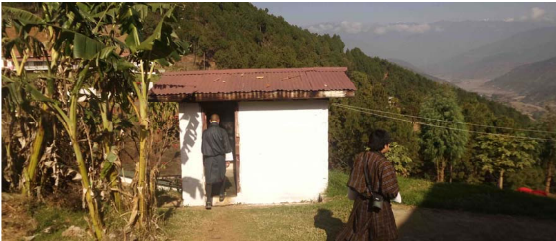
Figure Q2-02. Existing 1 indian-type restroom for all tourists and nuns at Sangchen nunnery ( Punakha )
