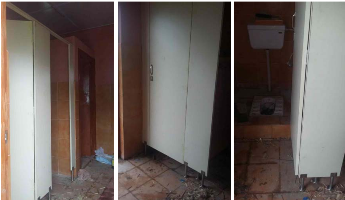
Figure Q3-34-38. Monitoring reports of Khewang Shedra restrooms construction.
