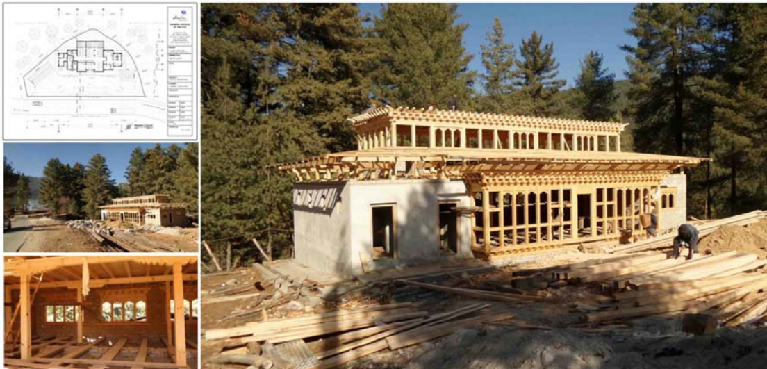
Figure Q5-71. Construction monitoring of tourists lounge at Tashichho Dzong.
