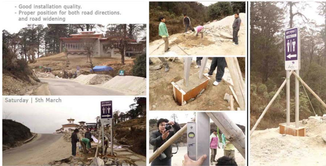
Figure Q2-138. Installation monitoring of Dochula restrooms signboard.
