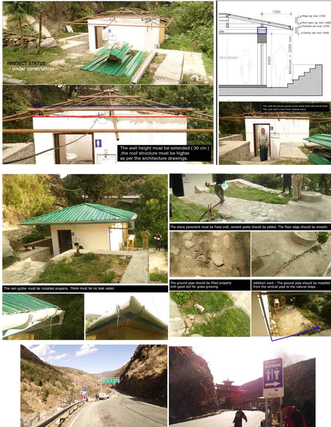
Figure Q3-39-42. Monitoring reports of Chuzom restrooms renovation and signboard installation.
