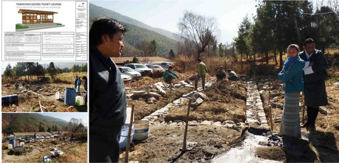
Figure Q5-70. Construction monitoring of tourists lounge at Tashichho Dzong.
