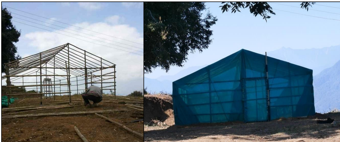
Figure 5. The second greenhouse is constructed with bamboo.
