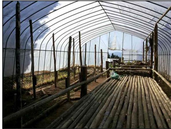
Figure 4. The first greenhouse after renovation and installation of bamboo shelves.
