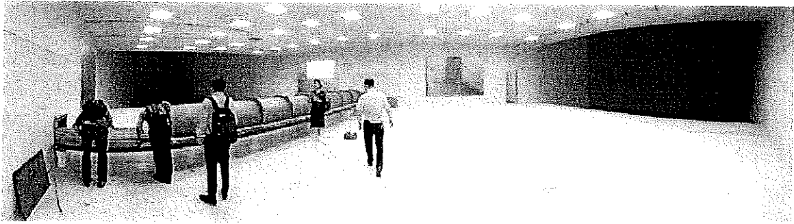
Wind tunnel system for high-speed railway
