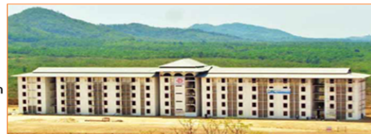
Building 501 (nearly fully completed)
