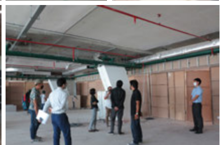
Renovation work by Maingan Furniture Supervision by Plan Architect
